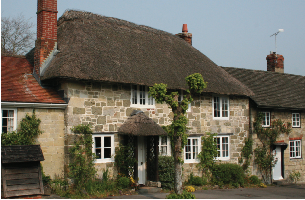
One of the few remaining thatched cottages in Hindon
