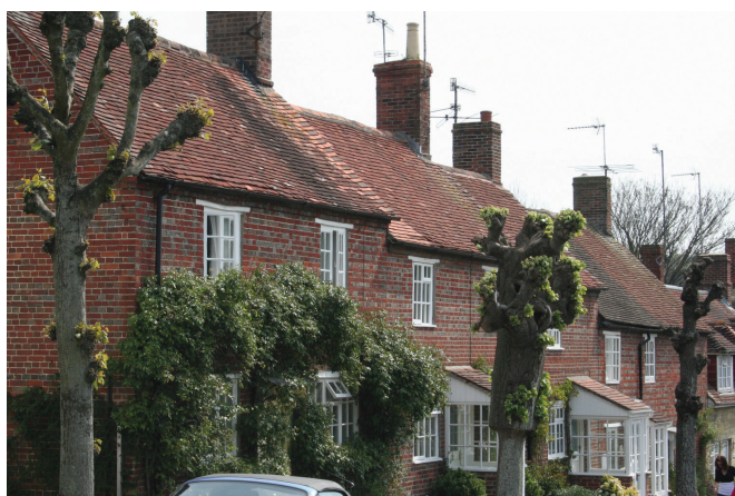
High Street roofline without dormers
