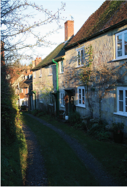
4. Looking East through Bakehouse Yard
