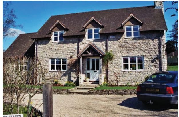
A Modern House with Traditional Features. Note the Open Porch and White-Painted Front Door and Dormer Windows. The use of White-Painted wood is attractive and sustainable. Use of stone, including for the dwarf garden wall, gives this house a very acceptable village appearance
